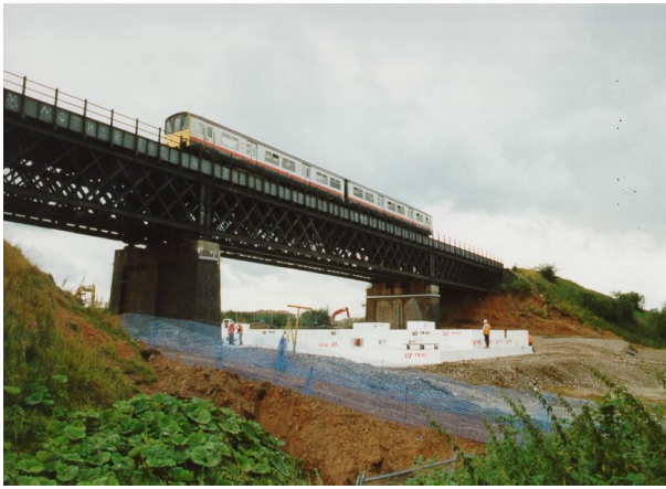
Figure 9. Continuing to place EPS blocks
