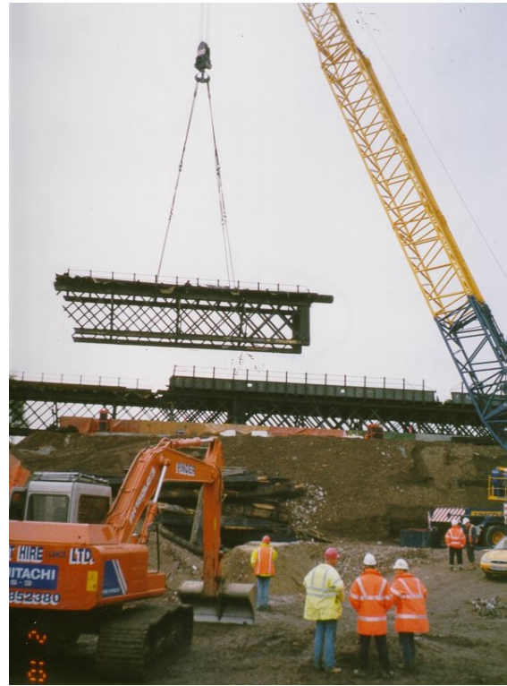
Figure 10. Possession works, demolition and removal of bridge deck
